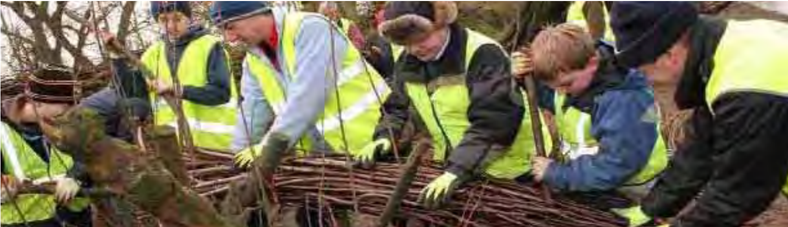
Environment Trust volunteers learning willow spiling to protect the riverbank at Kew. Photo courtesy Sarah Dixon
