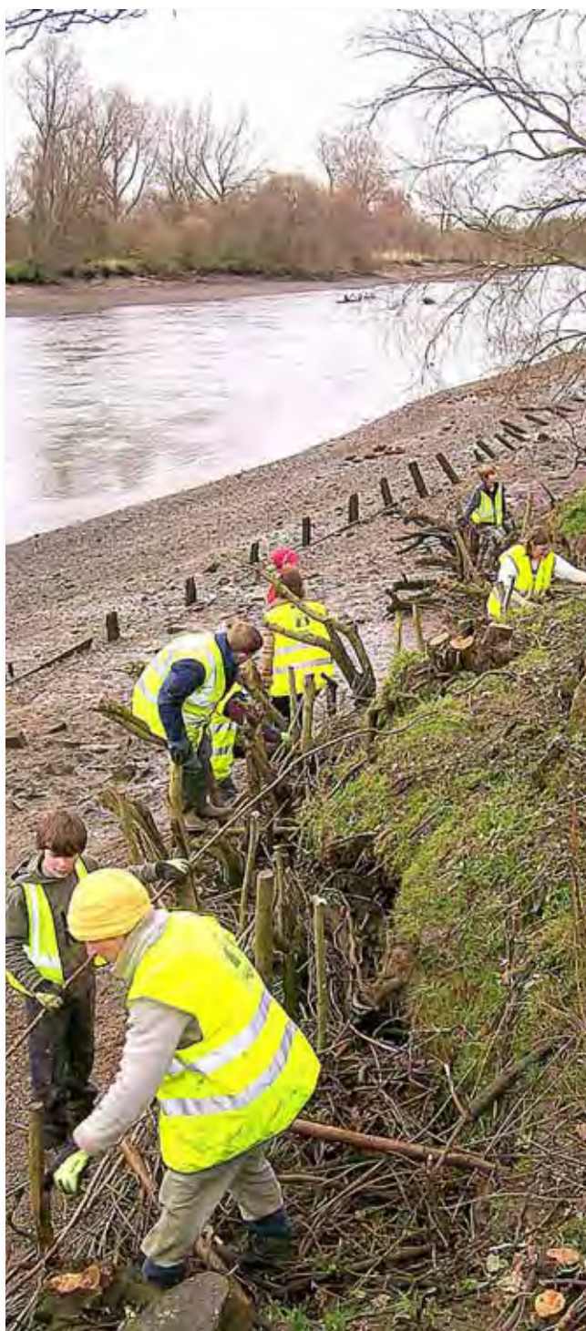
Willow spiling: a traditional conservation technique that Environment Trust volunteers have been putting into practice to protect the riverbank along Kew Reach
