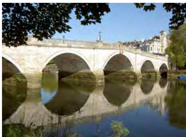
Richmond Bridge, built in the 1770s and still a vital link across the river
